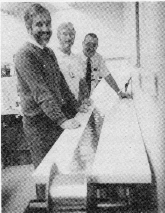
Dave Clouse, Jack Routsong and Eldon Andrews with foil being inspected for camber (curvature) parameter.
