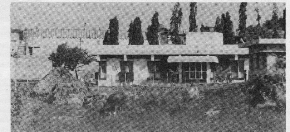
Control Room of the Godavari dam project.
