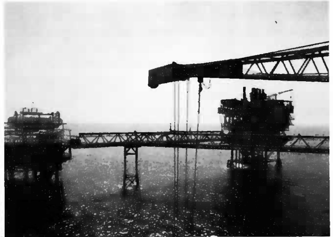
Chuck Berster was standing on Gas Lift Platform as he took this picture. At left is a Gas Extractor, atop the central production platform. The Gas Extractor recovers the natural gas previously injected into the well casing. At right is another platform where a contractor (Dugas) buys the recovered natural gas and sells it to its customers -- 60 miles away -- via a sub-sea pipeline.
