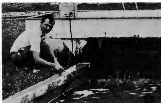
Bill Waggener with part of water pollution monitoring system at EMR-T's modern waste treatment plant.
