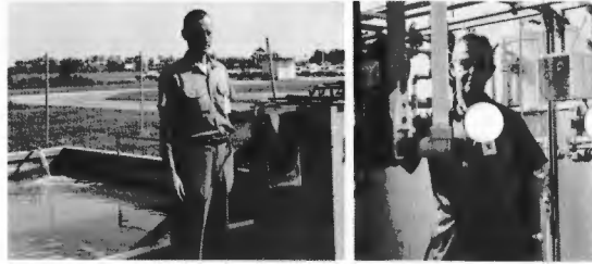
Harry Yates (left) holds stainless steel plate showing metal deposits removed from industrial wastes in our new chemical waste treatment plant. Right, Alden Brown gets ready to regenerate water filter system north of S-3 Building.
