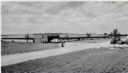
Original Production Building
