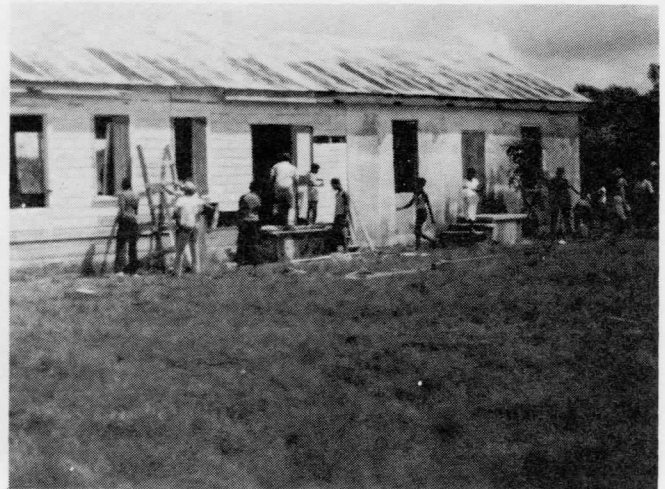
Starting the repairs on the Methodist Church building in Hattieville, Belize.
