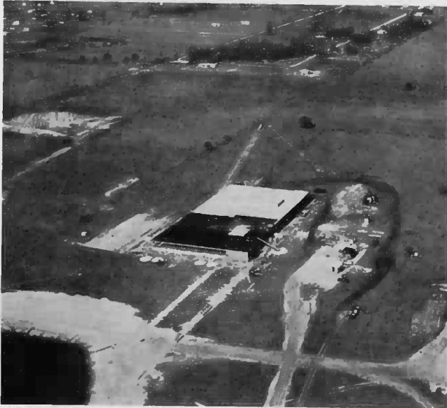
The Production Building, shown here under construction, was occupied in June, 1957.
