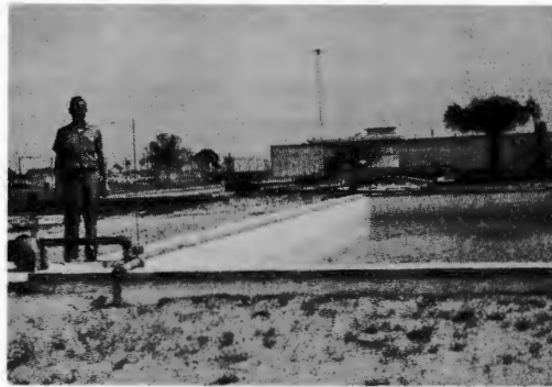
Harry Yates at new 40,000 gallon holding pond, part of EMR-T's advanced plant for safe chemical and sewage waste treatment.
