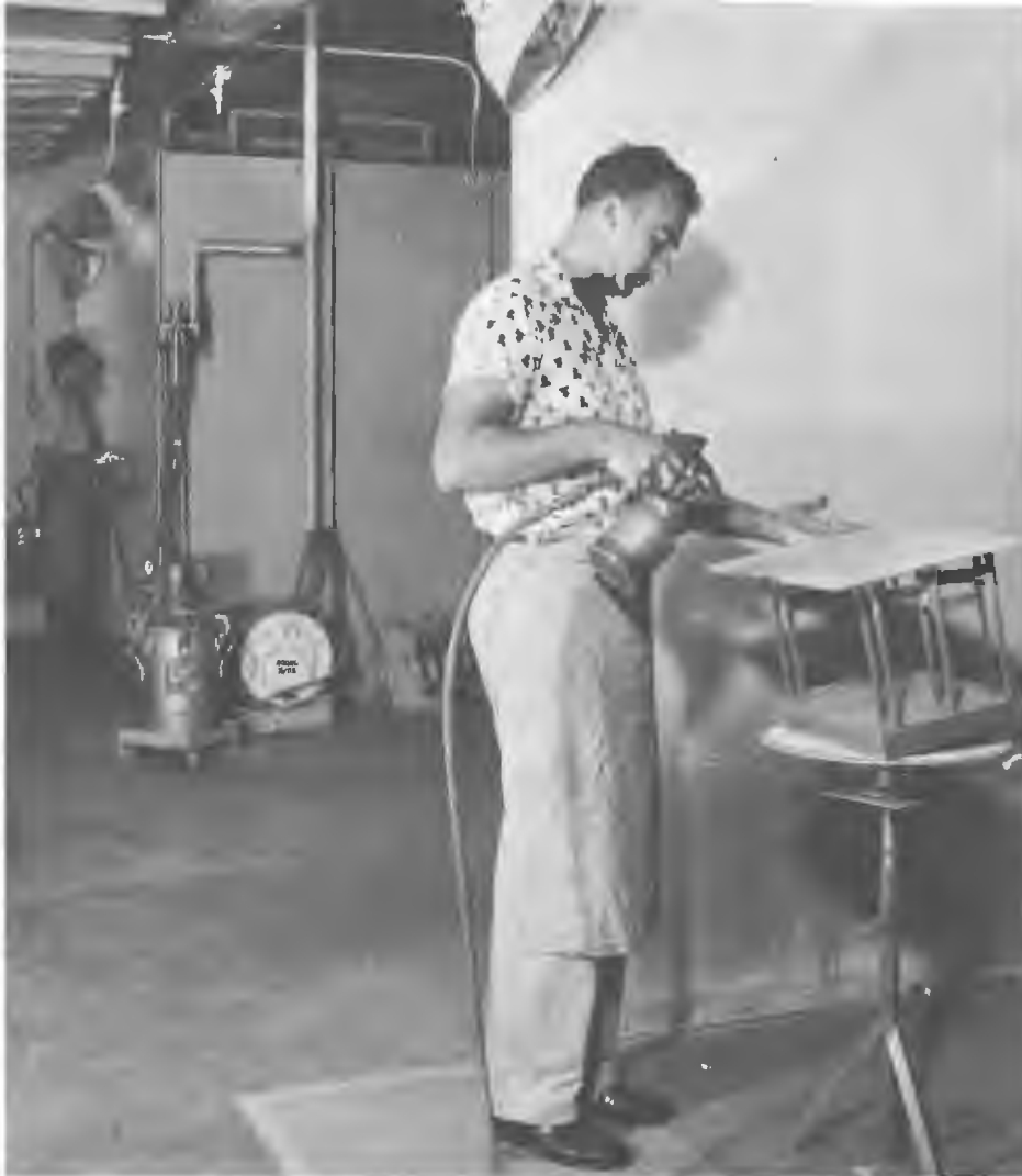
Spray painting in one of EMR's water-wash-equipped paint booths.
