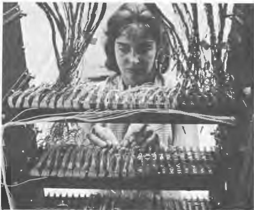
Nearly 10 miles of wiring are used in the assembly of each MSFTP-1 station
