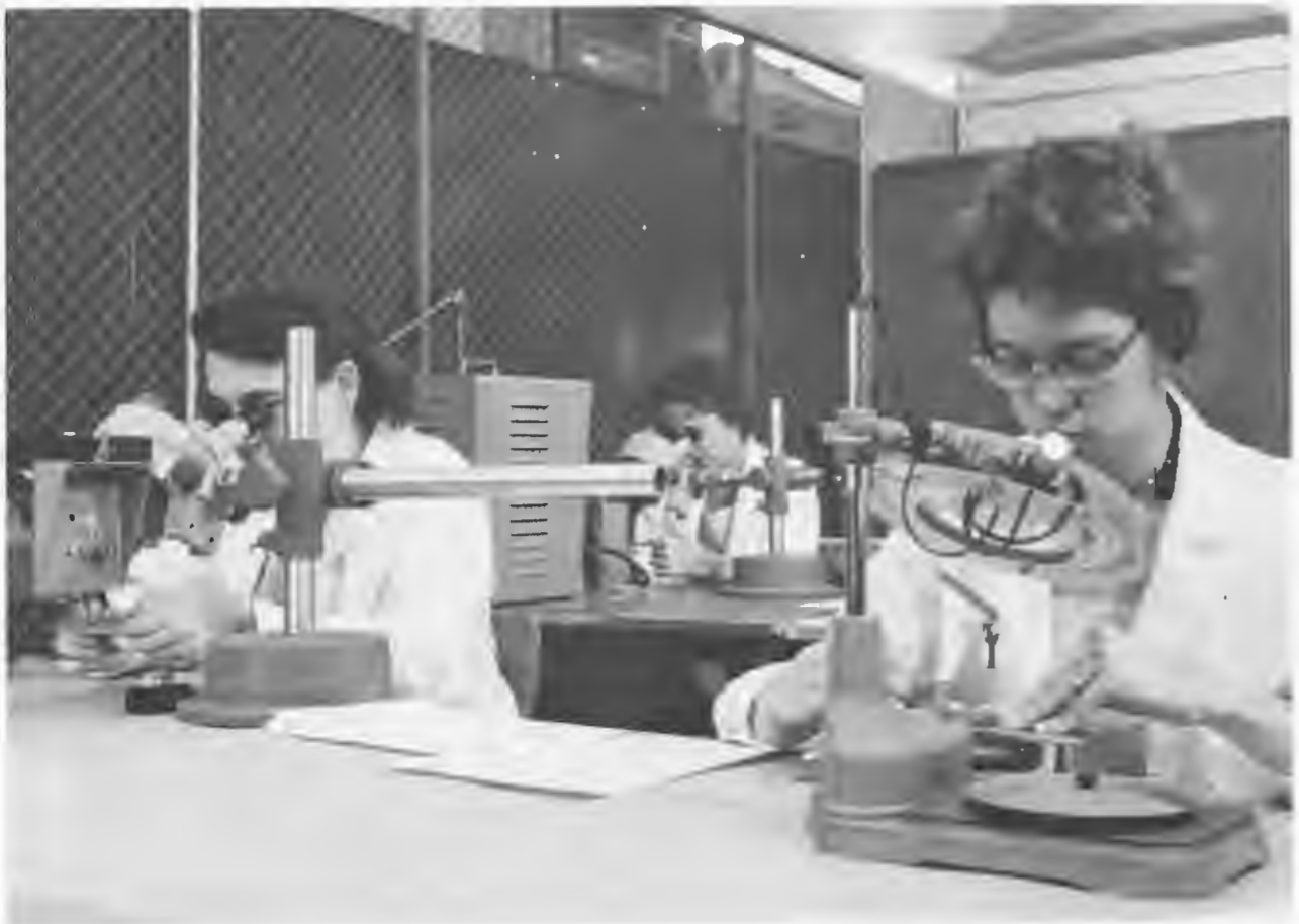
A portion of EMR assembly area where precision welding of miniature electronic subassemblies is accomplished
