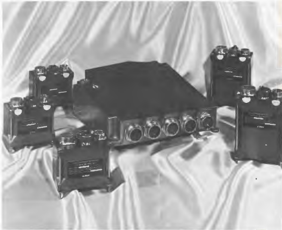
Gemini Spaceborne packages have 37,000 parts per cubic foot and consume approximately six watts.
